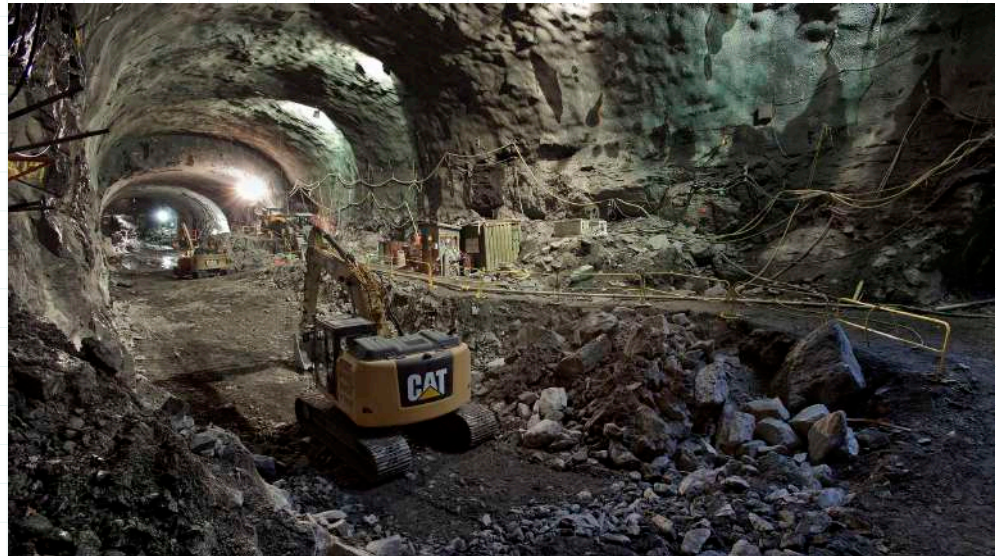
Second Ave Subway, New York
