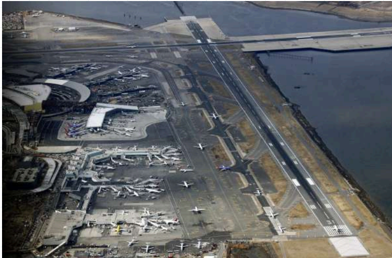
LaGuardia Airport Modernization, New York
