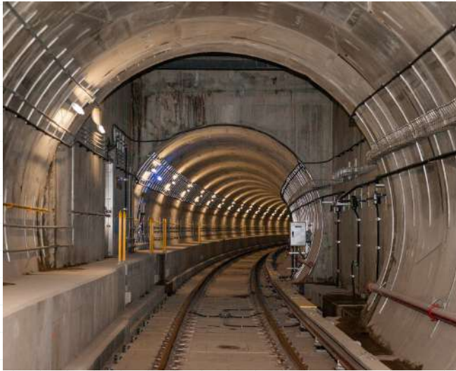
Toronto-York Spadina Subway Extension
